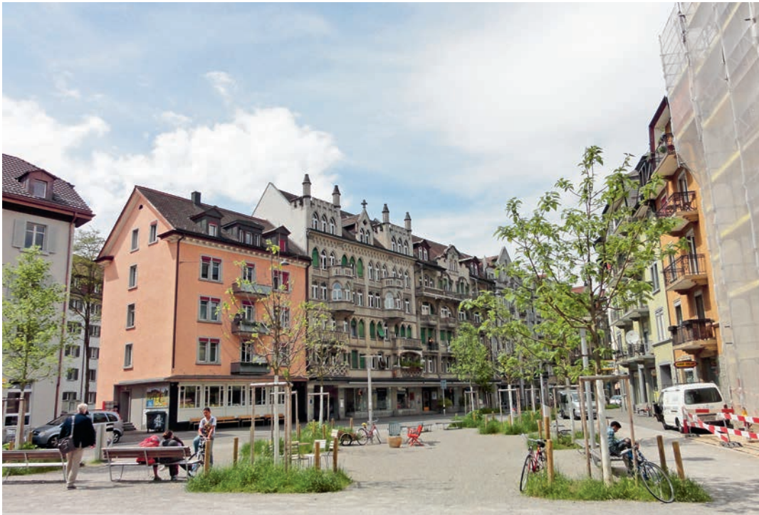
..... Above, Brupbacherplatz before the conversion.
