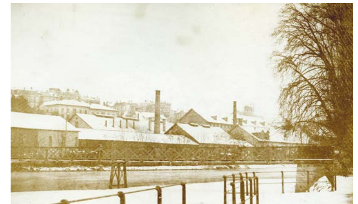
The former Escher-Wyss spinning mill on the river Limmat (Photo: Baugeschichtliches Archiv)
