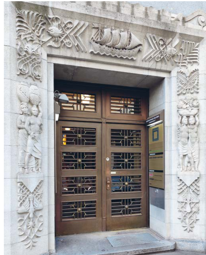
The entrance to the Sihlporte office building with colonial motifs (Photo: Curatorial team of the exhibition)
