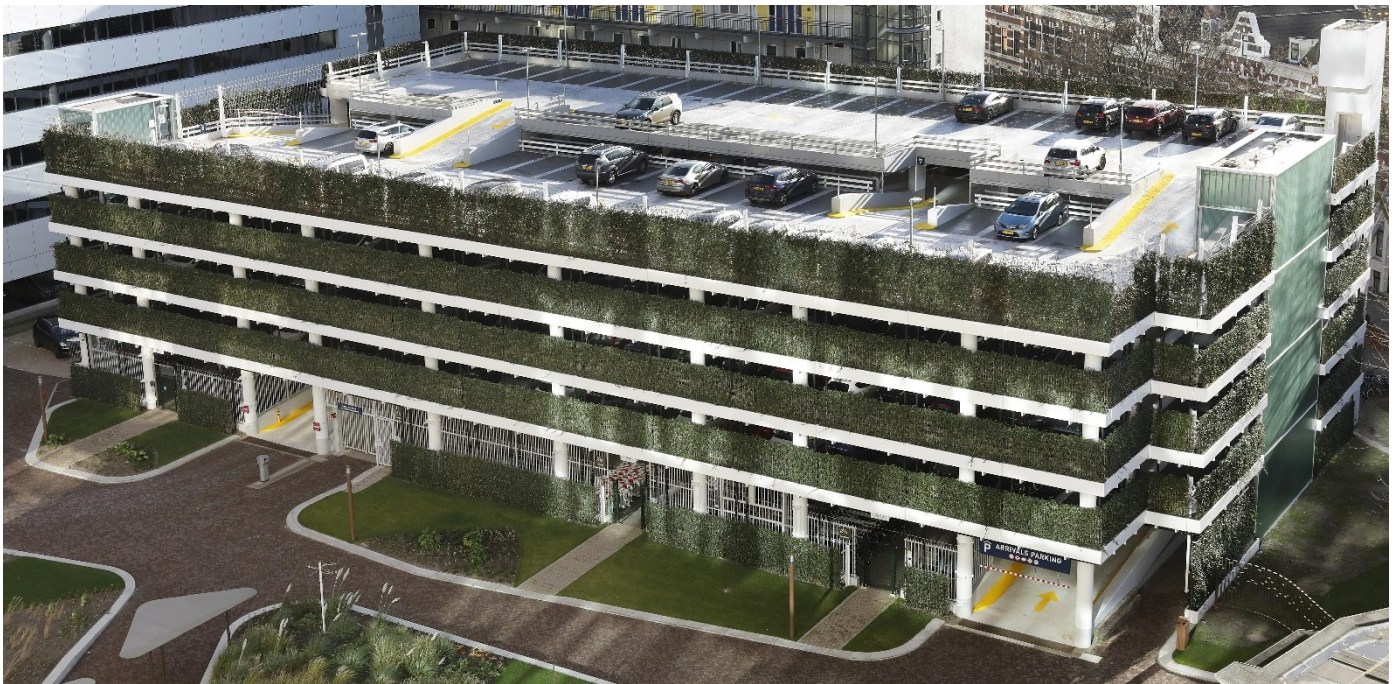
Gesamtansicht © WallPlanter green facade system: Parking Garage P-First, Rotterdam, The Netherlands
