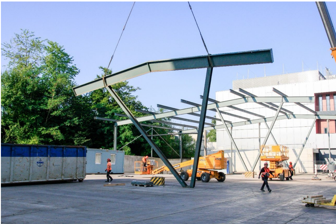
Abb.23 Demontage (© ZHAW IKE, 24.08.2024)
